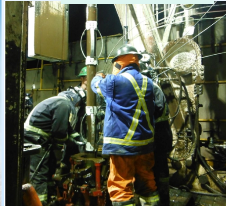
Casing Deployment Of Fiber Optic Lines
